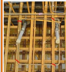
Setting concrete cover
