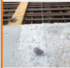
Aligning and fixing with wire
