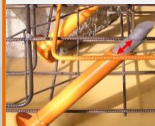
Screwing anchor rod
