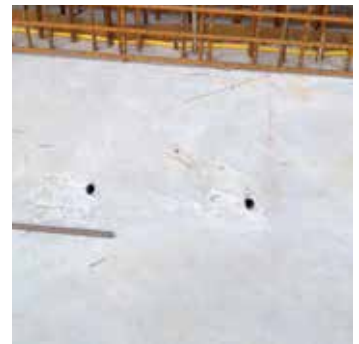
3. After concreting, pull out the foam plug.
