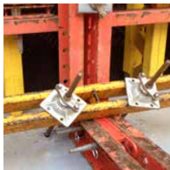
5. Anchor the formwork.
