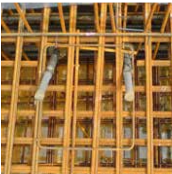
1. Align and tie the anchor.
