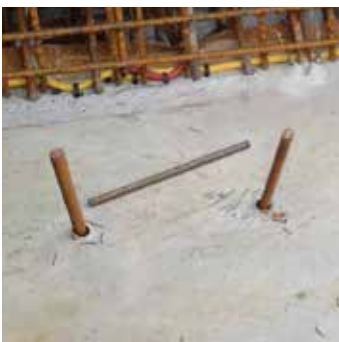
4. Screw in the anchor rods until the stop.
