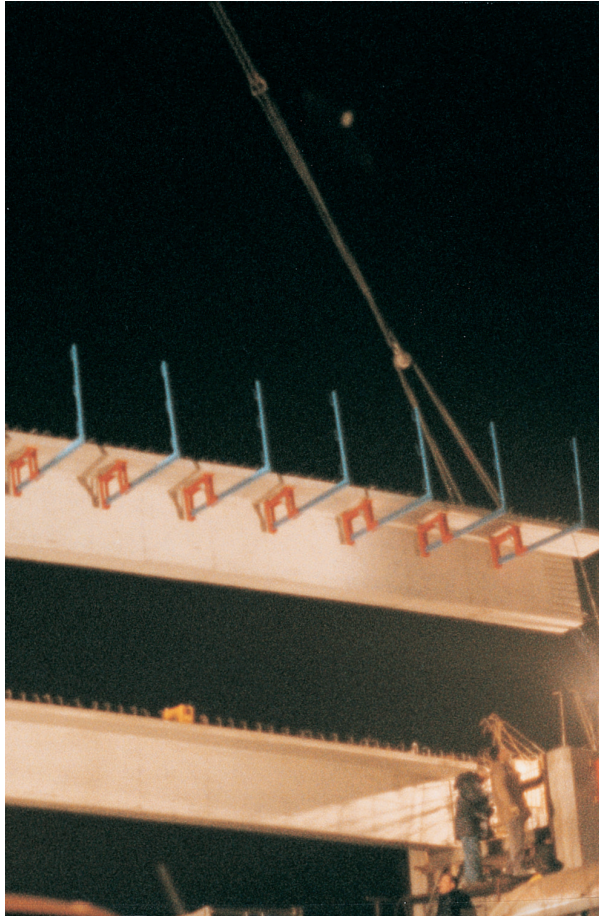
Cap bolt SF as cap formwork on abutments and support walls
