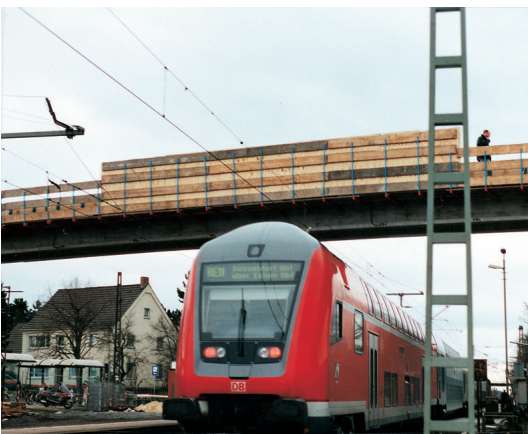
Cap bolt SF as a protective platform, in the railway driving area with baluster 180
