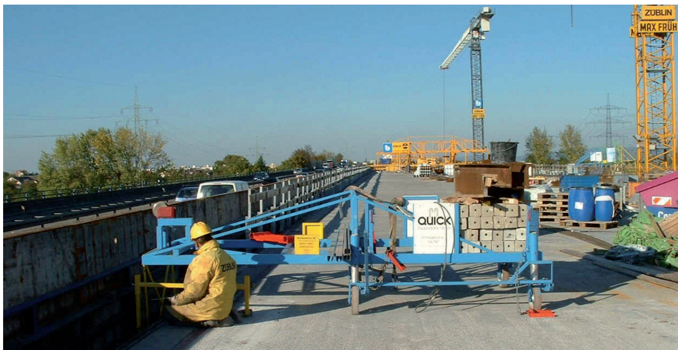
Assembly platform M 220 with a 220 cm cantilever arm
