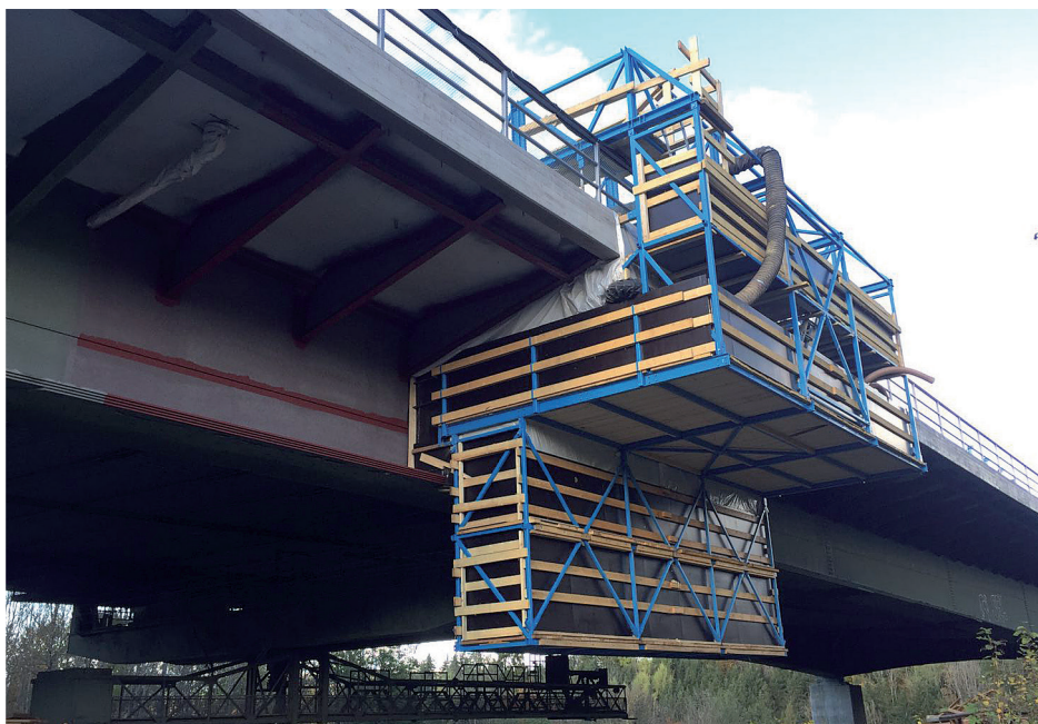
External working platform for corrosion protection of steel bridges
